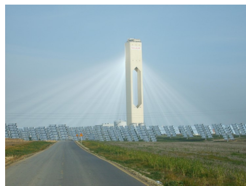
A concentrated solar power tower
